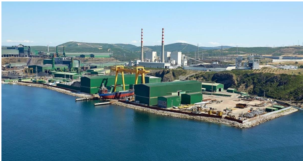
Figure 4: ICDAS Biga Steel Plant
