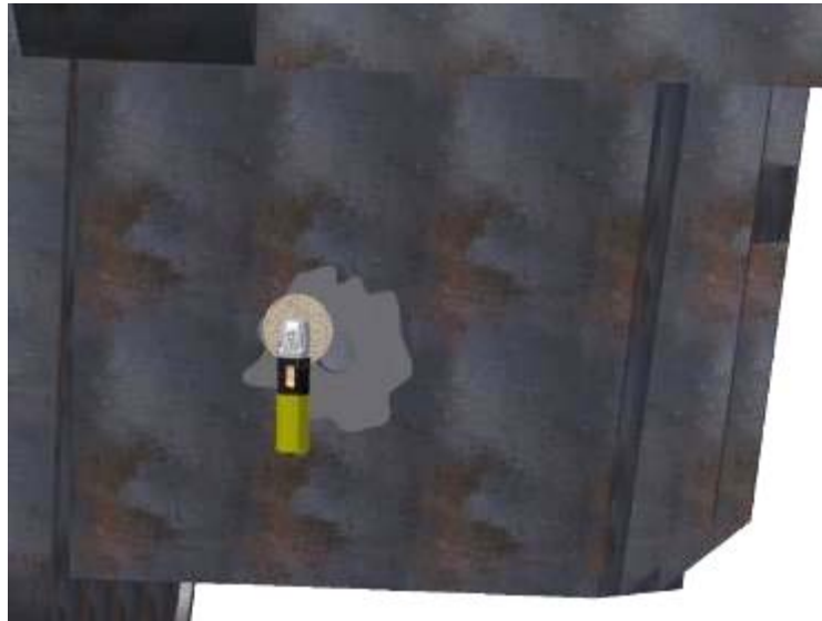
Figure 10 Grind the surface clean.
